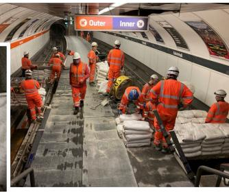
Gauge Clearance (lower levels of tunnel)
